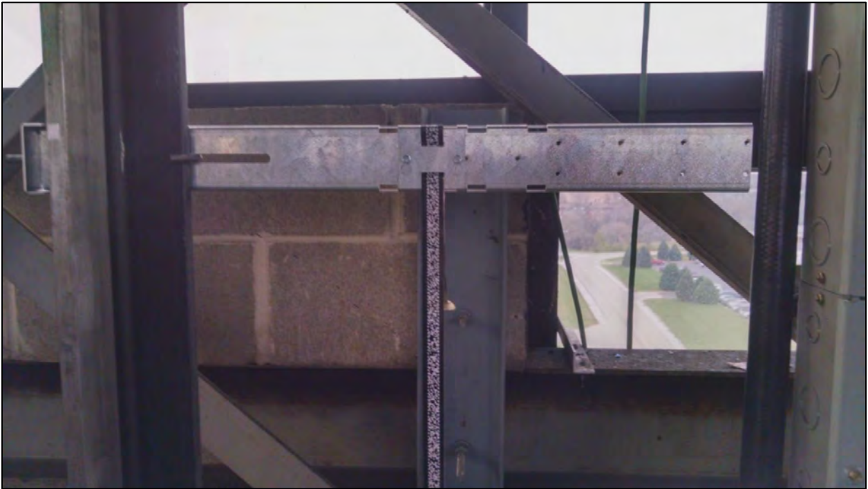
Figure 2-1: Encoded Tape Mounting – Top Bracket
