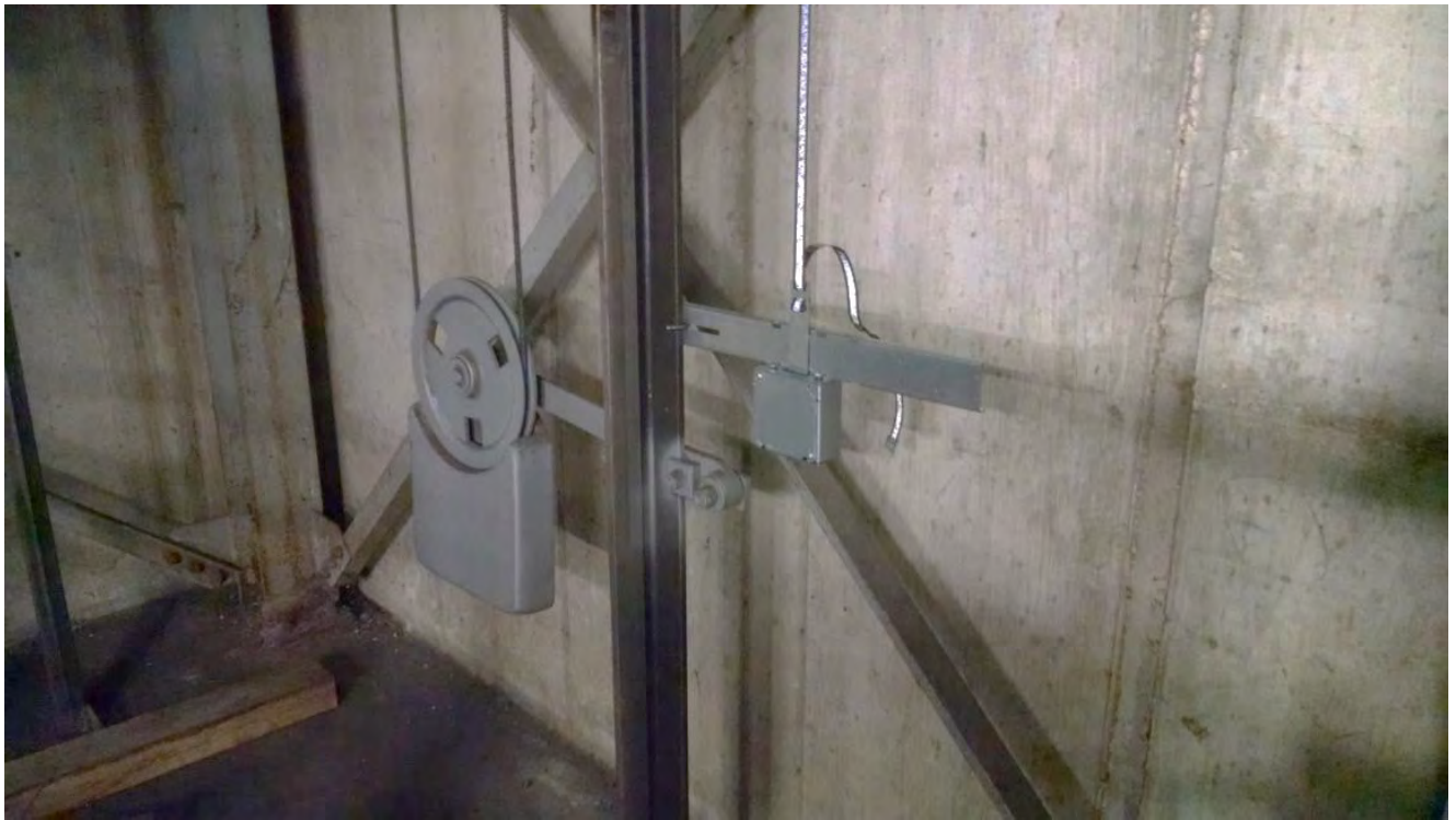
Figure 2-8: Encoded Tape Mounting – Bottom Bracket
